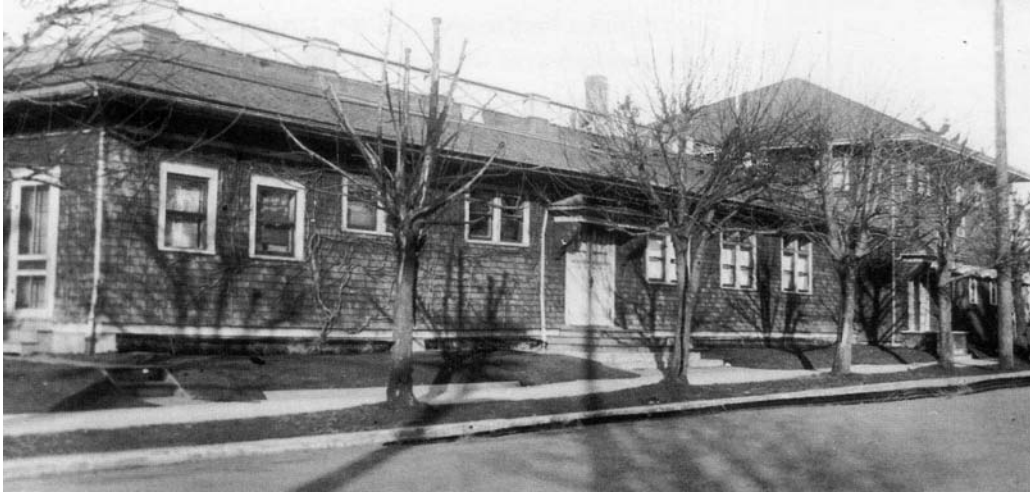
Clubhouse with 1912 addition
