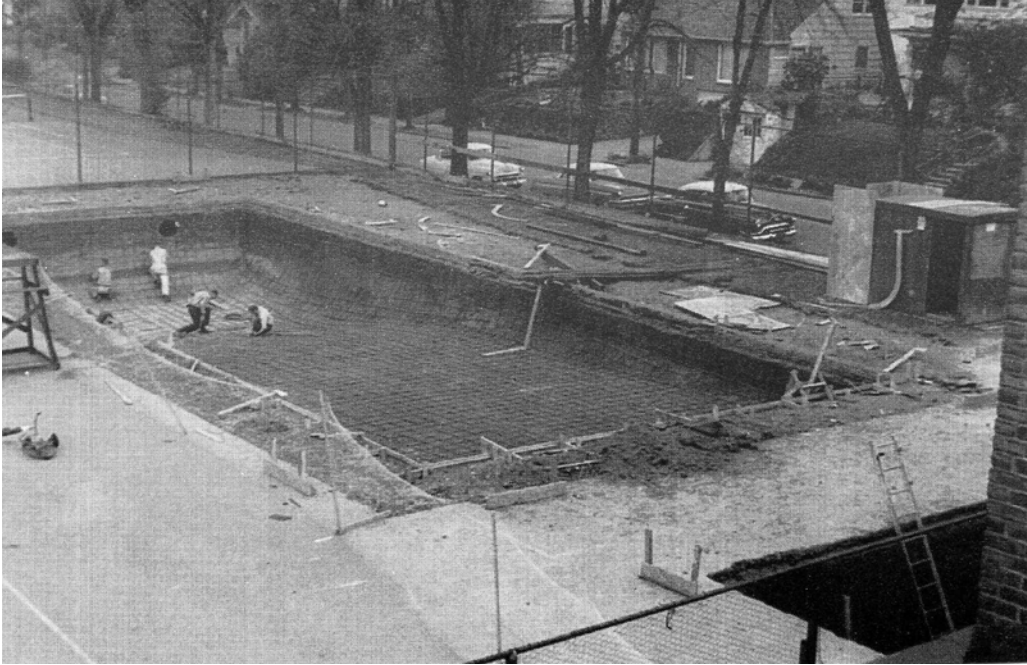
Construction of the pool, 1957
