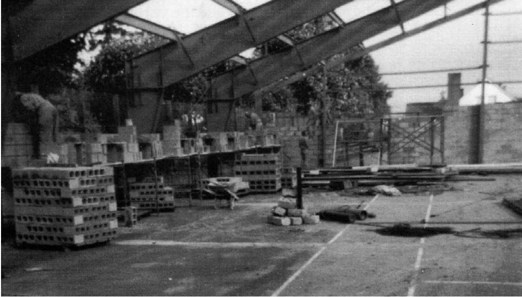
Construction workers covering the first two courts, October 1965
